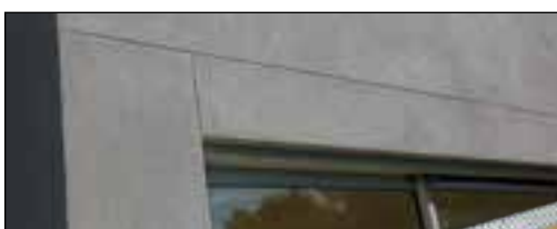
Figure 3.4.1 Neat finish of horizontal joints
